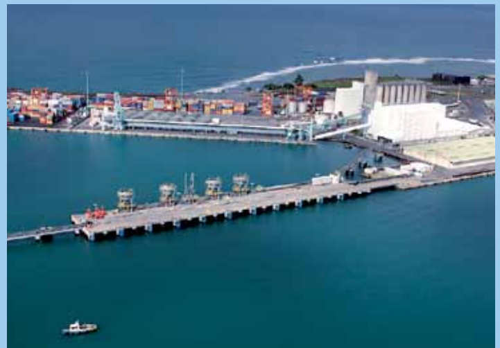
The Mole B at the Port of Toamasina, built by Ambatovy
